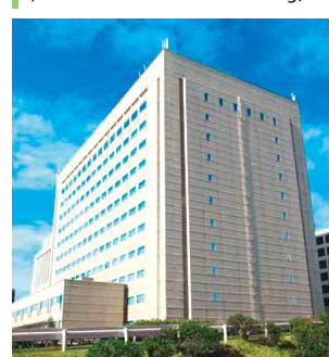
Sumitomo Shoji Senri Building (Data Center / Office Building)
