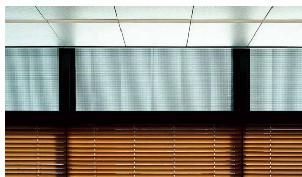
Window surface in the natural lighting system
