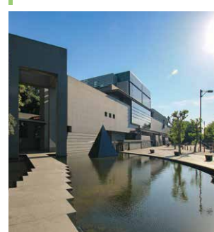
Fuchu Data Center
