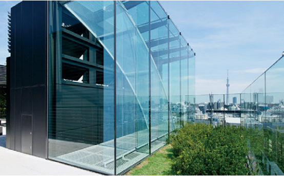
Natural ventilation (rooftop solar chimney)
