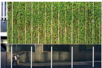
Greening of Walls
