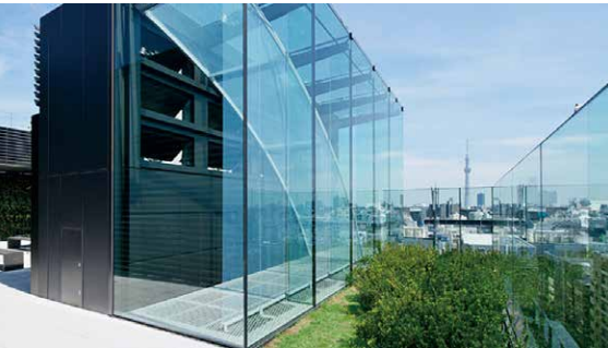
Natural ventilation (rooftop solar chimney)
