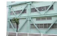
An example of reinforcement work
