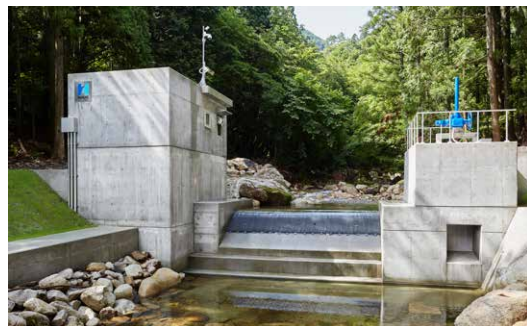
Kamogawa Small Hydroelectric Plant
