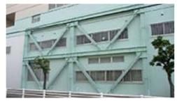
Seismic reinforcement using steel brace (LICOPA Tsurumi)
