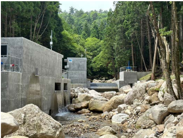
Kamogawa small hydroelectric plant water intake
