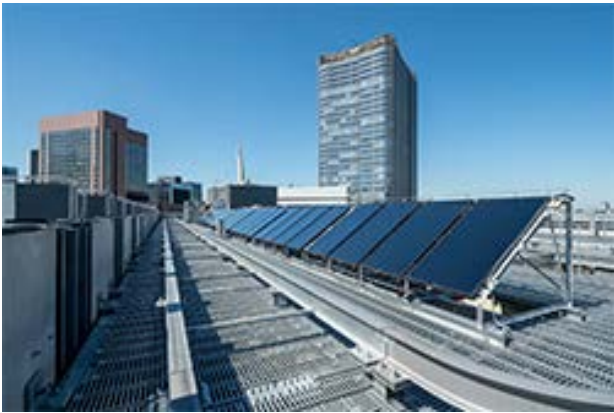
Solar heat collection panels (HULIC SQUARE TOKYO)
