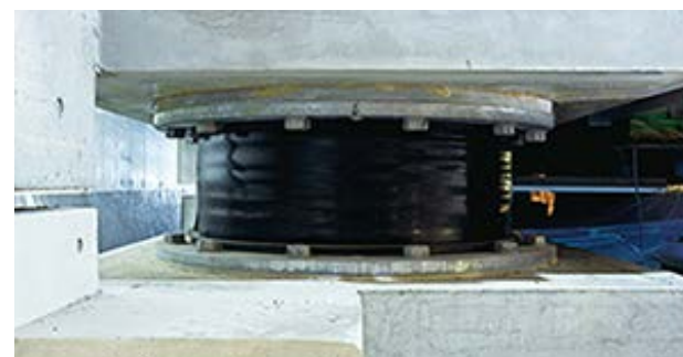
Earthquake-absorbing equipment
