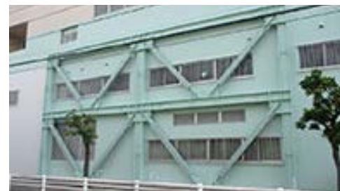
Seismic reinforcement using steel brace (LICOPA Tsurumi)
