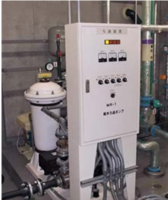
Rainwater filtration equipment
