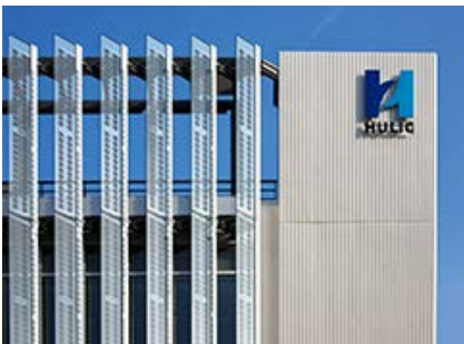
The exterior wall with photovoltaic panels (Hulic Ogikubo Building)
