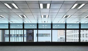
Natural lighting louvers and LED lighting (HULIC Head Office Building)
