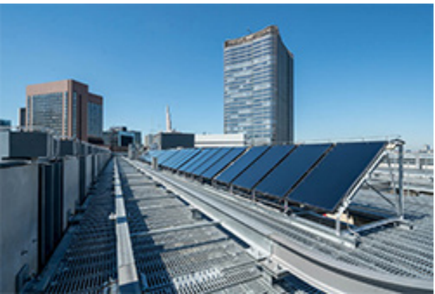
Solar heat collection panels (HULIC SQUARE TOKYO)
