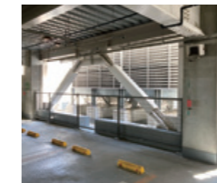
An example of reinforcement work
