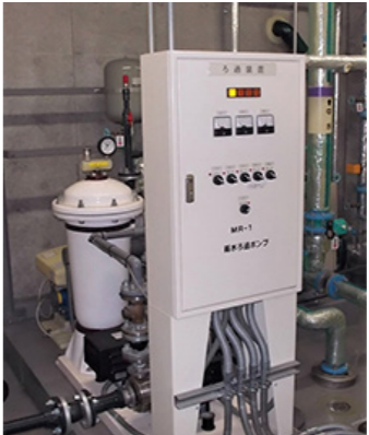
Rainwater filtration equipment
