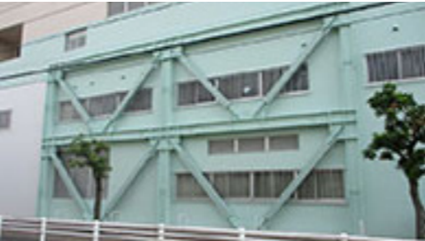
Seismic reinforcement using steel brace (LICOPA Tsurumi)
