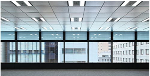
Natural lighting louvers and LED lighting (HULIC Head Office Building)
