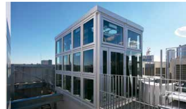
Rooftop solar chimney (Hulic Shinjuku Building)
