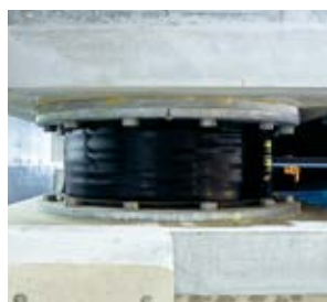
Earthquake-absorbing equipment
