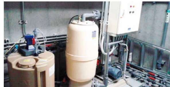
Rain water reutilization equipment at Hulic Setagaya
