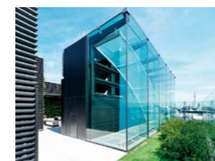
Rooftop solar chimney (Hulic Head Office Building)
