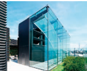
Rooftop solar chimney (Hulic Head Office Building)
