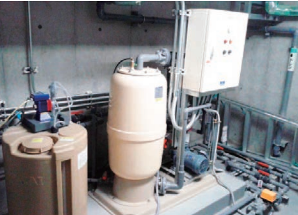
Rain water reutilization equipment at Hulic Setagaya
