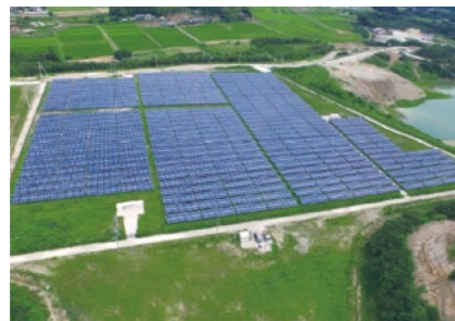
Hirono Town Solar Power Plant
