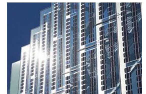
The exterior wall with photovoltaic panels (Hulic Ogikubo Building)
