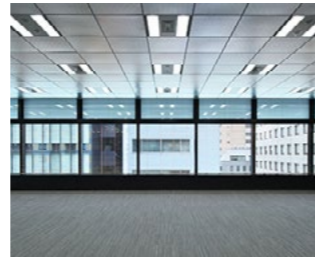
Natural lighting louvers and LED lighting (HULIC Head Office Building)
