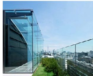
Rooftop solar chimney (HULIC Head Office Building)
