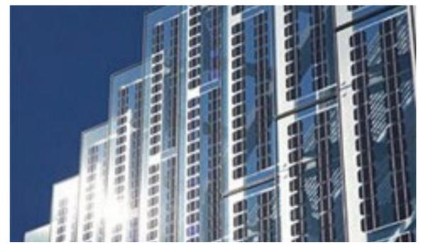
The exterior wall with photovoltaic panels (Hulic Ogikubo Building)
