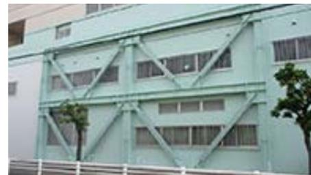
Seismic reinforcement using steel brace (LICOPA Tsurumi)
