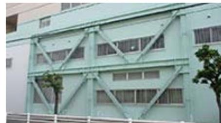
Seismic reinforcement using steel brace (LICOPA Tsurumi)
